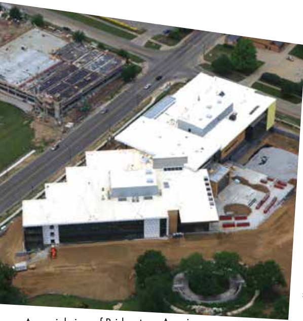
An aerial view of Bridgestone Americas Technical Center's roof system
