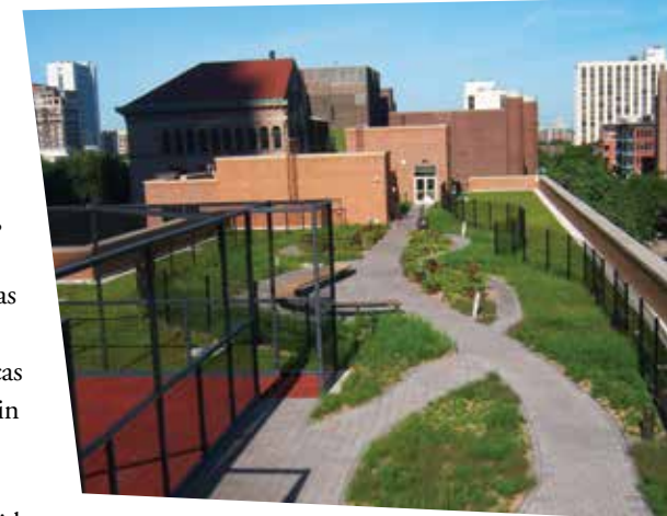
View of Ogden International School of Chicago's vegetative roof system from the building's northeast corner
